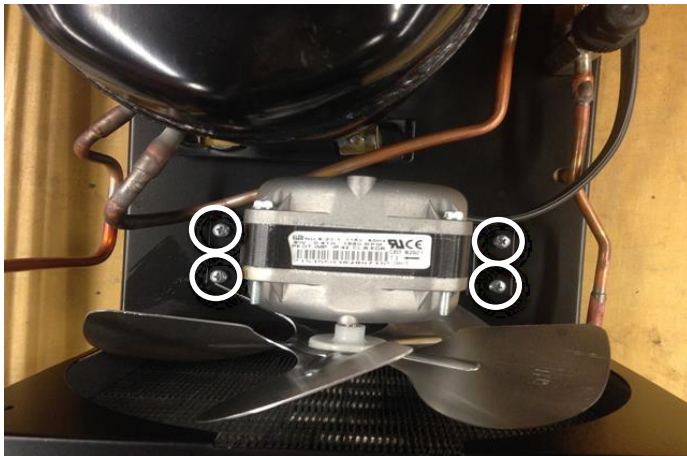
Figure 6-9. Fan Mounting Hardware
