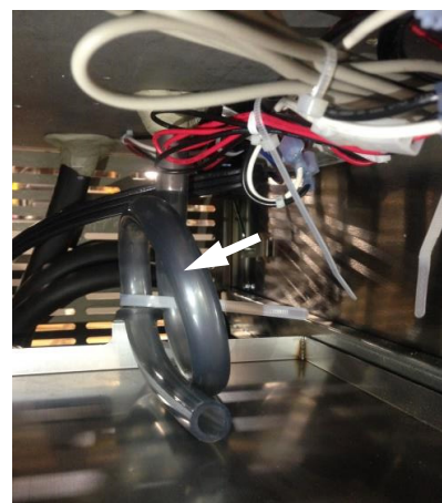
Figure 6-3. Evaporator Condensate Trap
