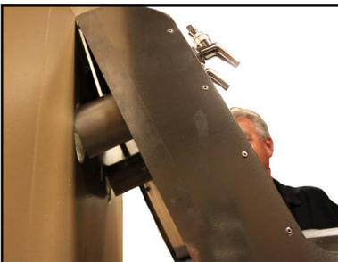
10. Insert the hang tab at the top edge of the dispenser into the hang track on the wall.
