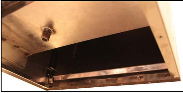
11. Secure the bottom edge of the dispenser to the wall. Use appropriate anchors for the type of wall you're attaching the dispenser to. Ideally, drive screws into wall studs where possible.
