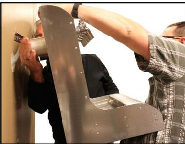
9. Feed hose duct and beverage leads through the corresponding 3-1/2" to 4" holes drilled through the cooler wall.
